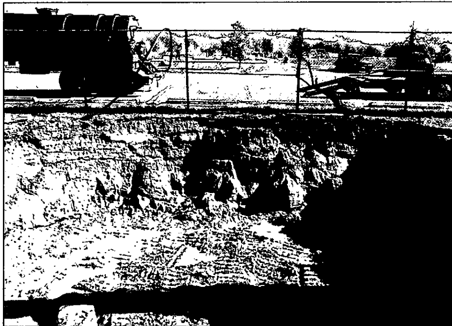
Photo #8: View of east wall of excavation, facing east.
